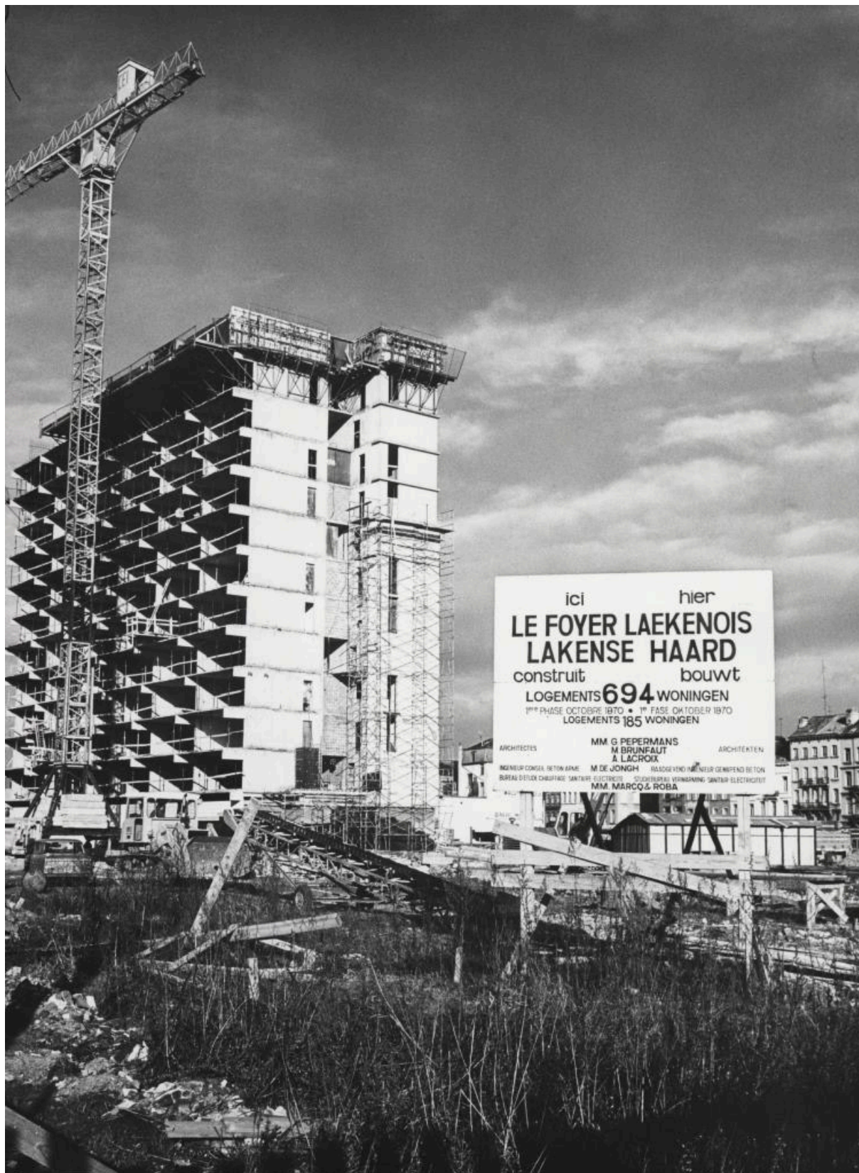
Construction of the blocks of the foyer Laekenois
